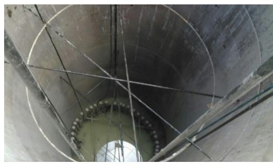
120-inch Diameter Steel Temporary Casing
