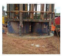
O-Cell assembly at tip of reinforcing cage
