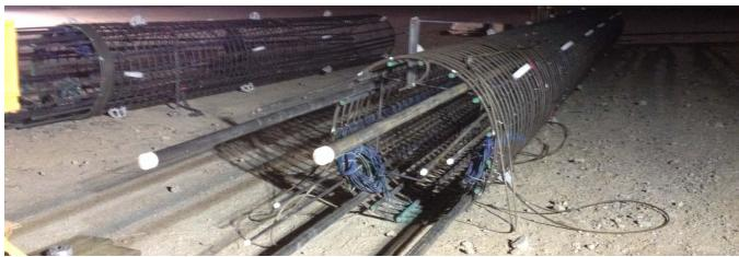
Shaft reinforcement with O-cell assembly.
